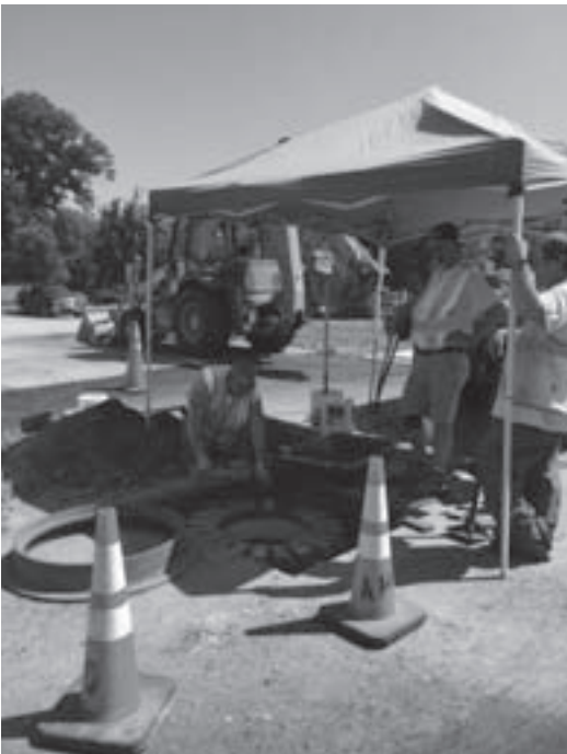
Raising a drainage manhole on Ferry Street
