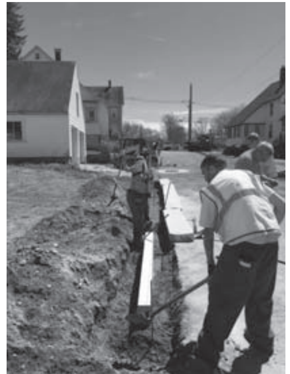
Installing a new curb on Reynolds Avenue
