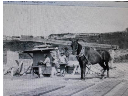
Head & Bailey Brick Yard
