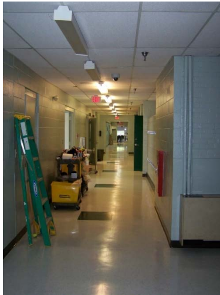
Typical corridor lighting
