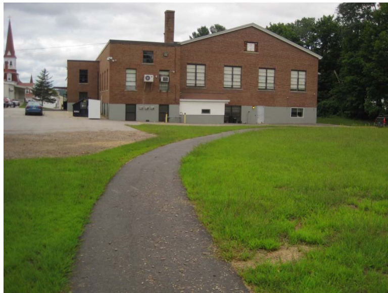
East elevation with Church steeple on left
