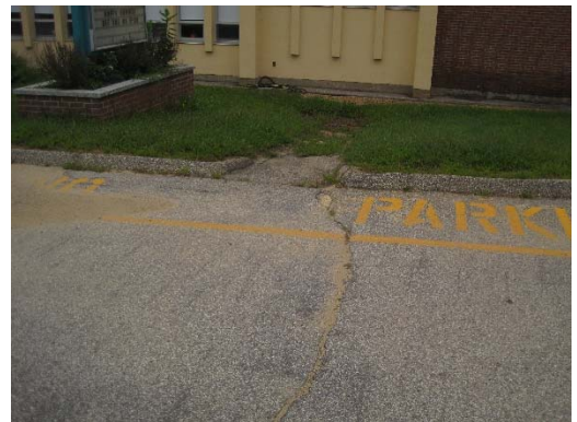
Curb cut that leads to catch basin
