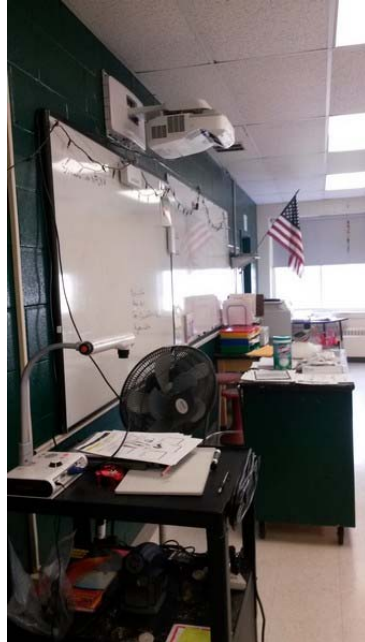
Wall mounted projector with marker board
