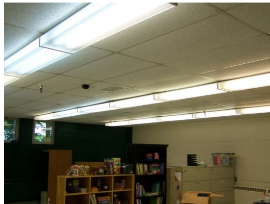
Typical classroom with surface mounted lighting
