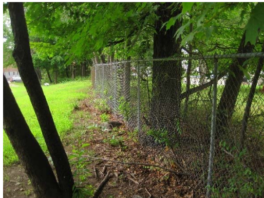
Northern perimeter fence in good condition
