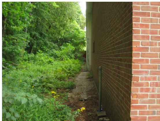
North elevation of 1988 addition
