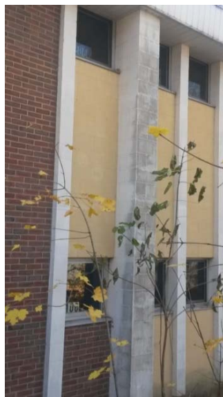
Original 1973 two story north elevation original windows
