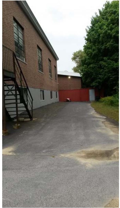
North elevation with 1973 building beyond
