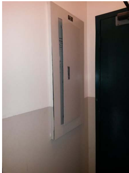
Panelboard LPG is located in an egress stair at the music classroom
