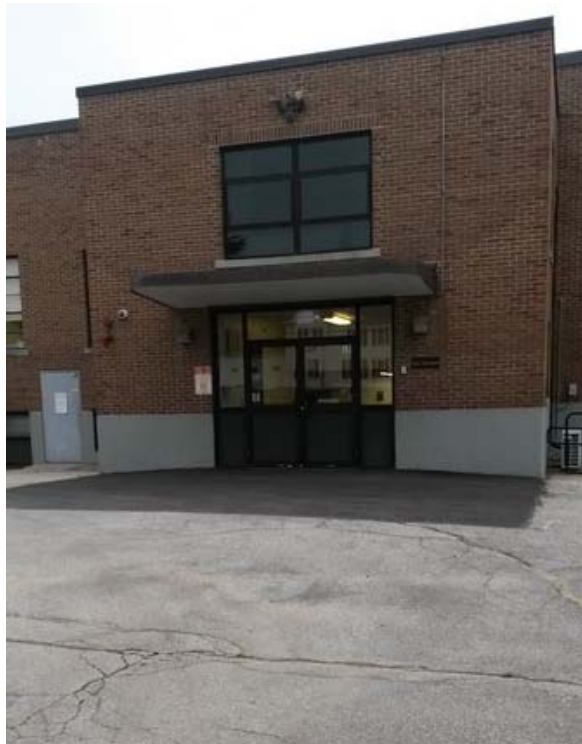
Front south elevation - Main entrance through Lobby #117 to Gym and Cafeteria
