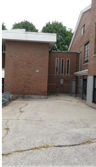
Connector elevation with original 1954 Gym & Cafeteria on the right
