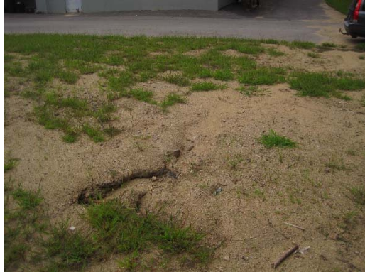
Erosion area noted to the northeast of the building
