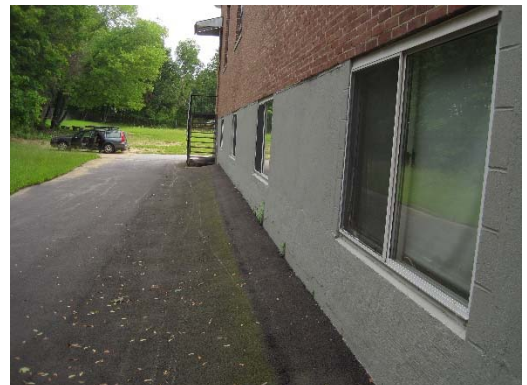
Pavement north of school (looking east)
