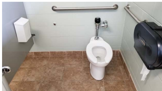
Second Floor Girls ADA Stall
