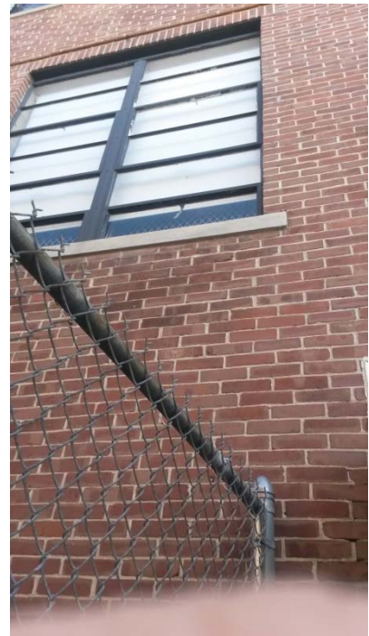
Original 1954 examples at Gymnasium with steel frame single pain windows
