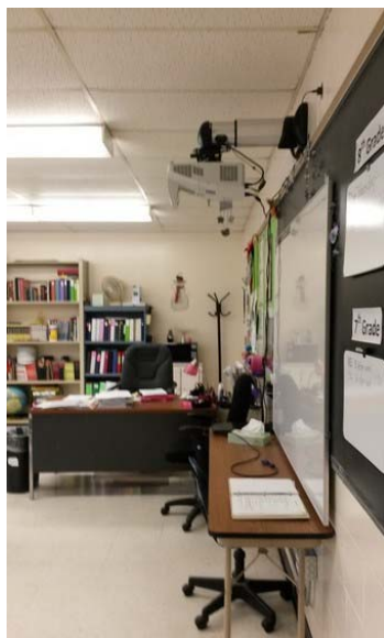
Projector with marker board mounted over existing chalk board
