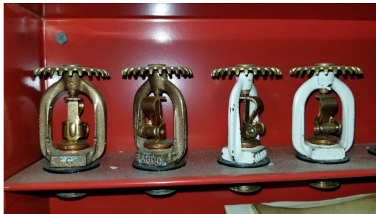
Spare Sprinkler Cabinet
