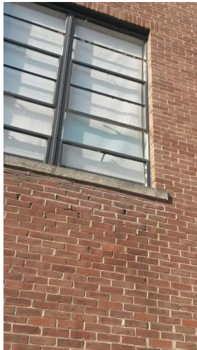
Original 1954 examples at Gymnasium with steel frame single pain windows
