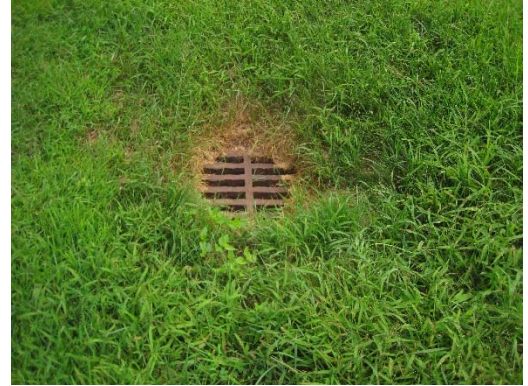
Catch basin within the vegetated area near building
