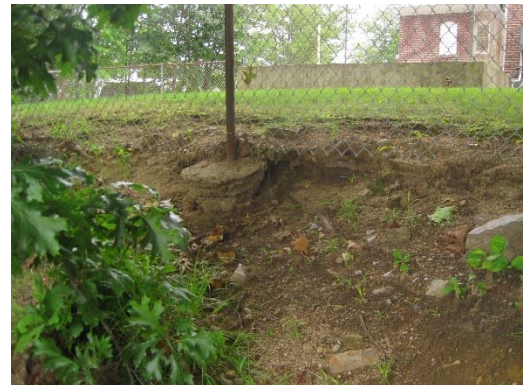
Exposed concrete post foundation at west perimeter
