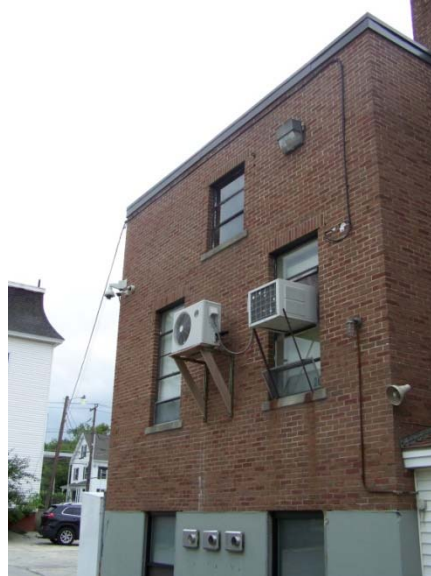
Building mounted lighting fixture
