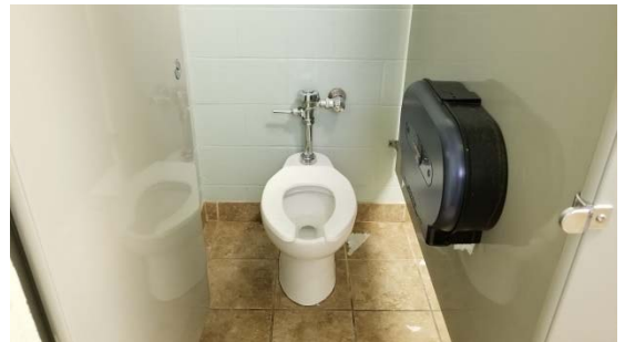
Second Floor Boys Typical Stall
