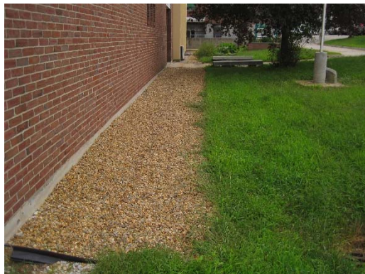
Perimeter drain along southern wall of western building
