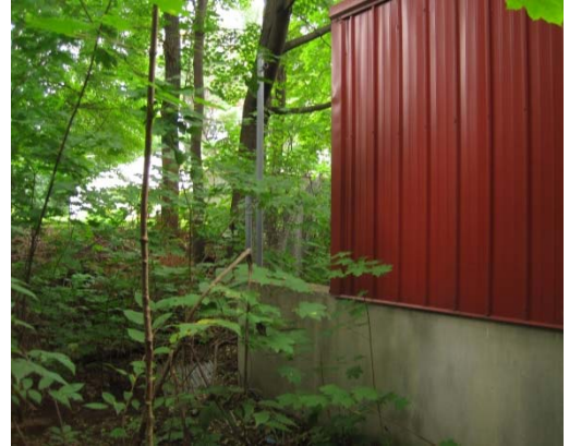
Red storage addition by connector reduces site access to less than 20 feet
