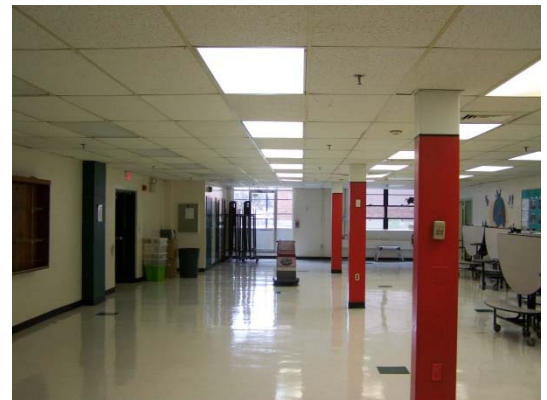
Recessed / flush lighting, cafeteria
