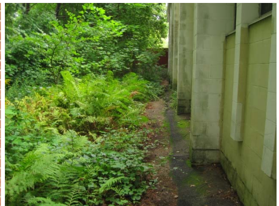
North elevation of original 1973 building
