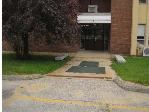
Trench drain at curb cut leading to entrance
