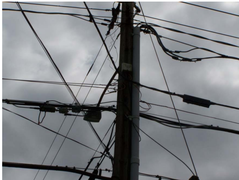
Building fire alarm connection to the city loop at School Street
