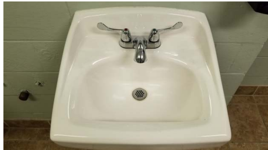
Second Floor Boys ADA Lav
