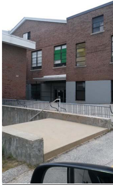
West elevation of 1954 original building with corner of 1973 building on the left
