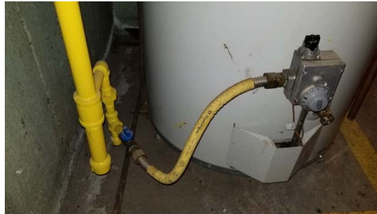
Existing Natural Gas Fired Water Heater
