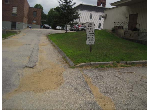
One-way signage heading eastbound on access way
