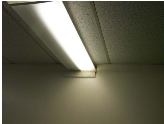
wall built around lighting fixture run
