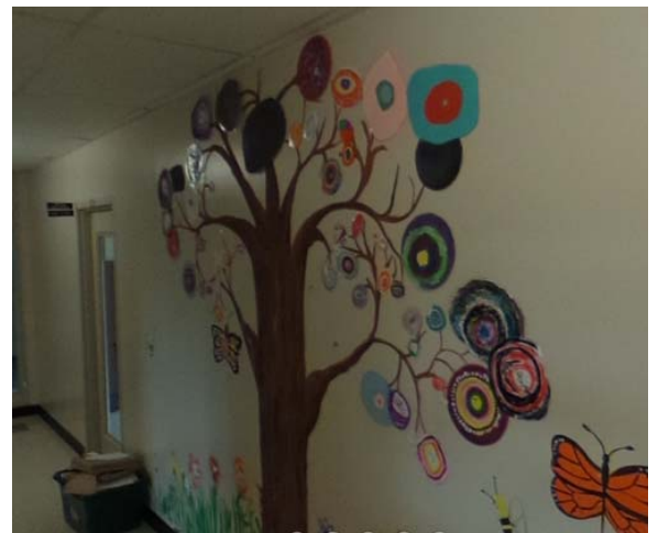
Gypsum wall board
