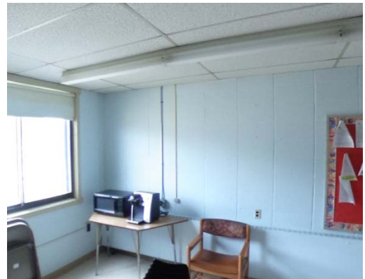
CMU wall - stacked bond coursing
