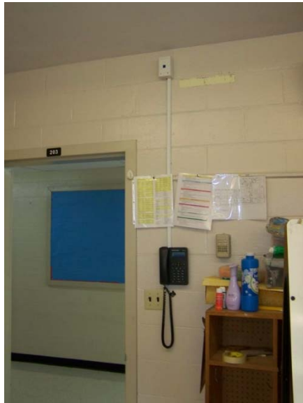
typical classroom, phone at door
