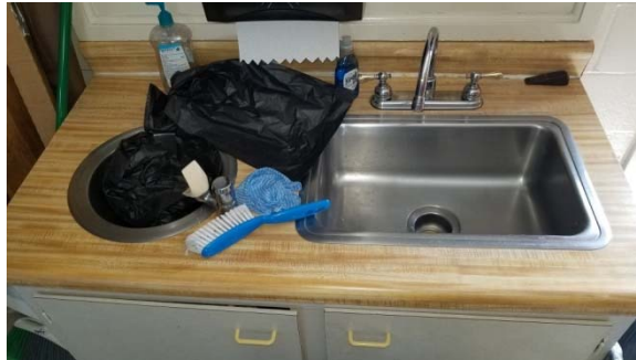
Typical Classroom Sink with Bubbler
