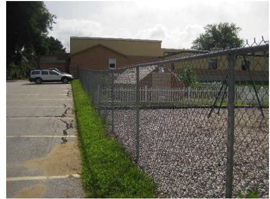
Northern perimeter fence in great condition
