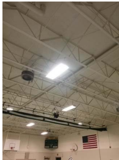
Exposed structure and deck
