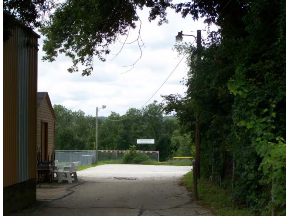
pole mounted flood lighting, utility company leased lights to ball fields, right side of building
