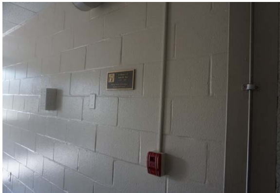
CMU wall - running bond coursing
