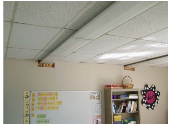
another example of wall built around lighting fixture run
