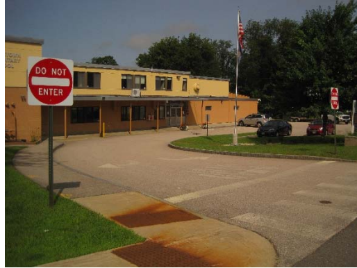
ADA ramps and detectable warning plates
