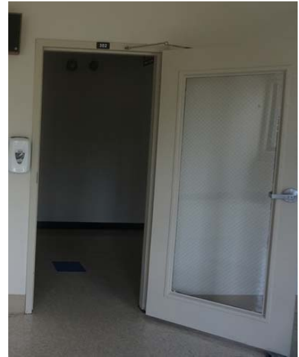
Typical hollow metal door with full glass
