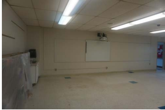
Acoustical ceiling tiles
