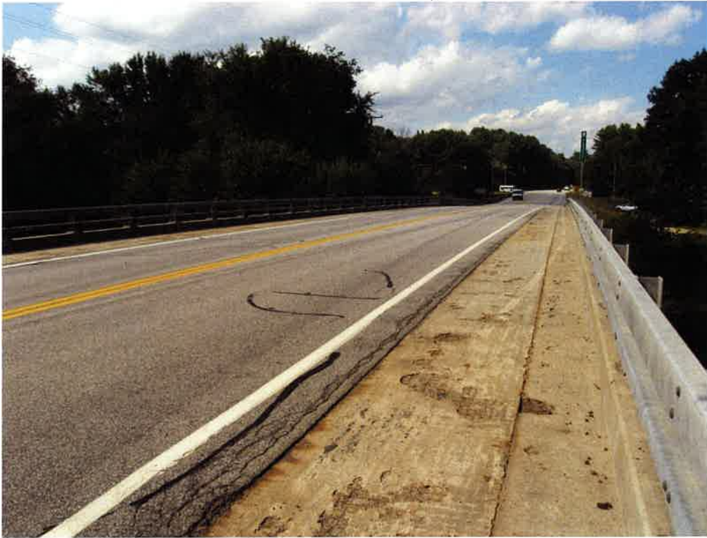
3. Allenstown Bridge No. 107/098, south railing along roadway, facing north. 08/15/2019.
