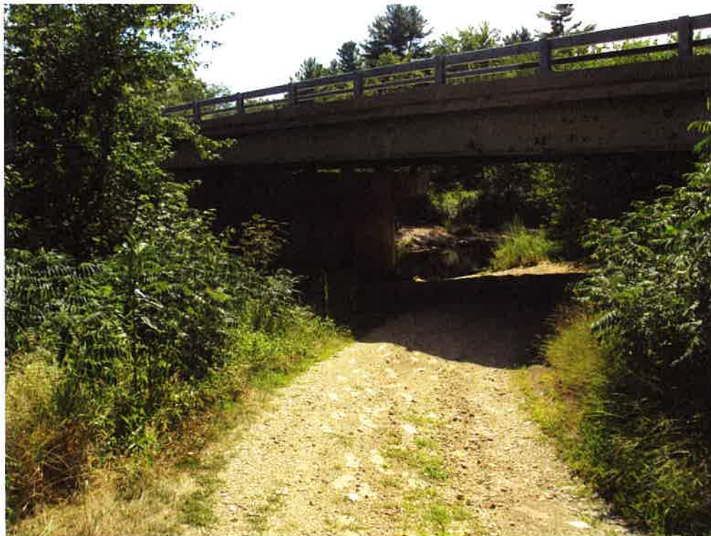
2. Allenstown Bridge No. 107/098 profile, facing southwest. 08/15/2019.
