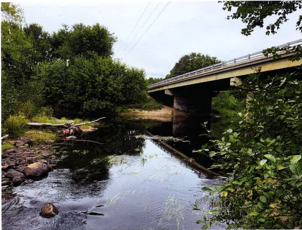
12. View north along the western side of Allenstown Bridge No. 107/098. 09/06/2019.
