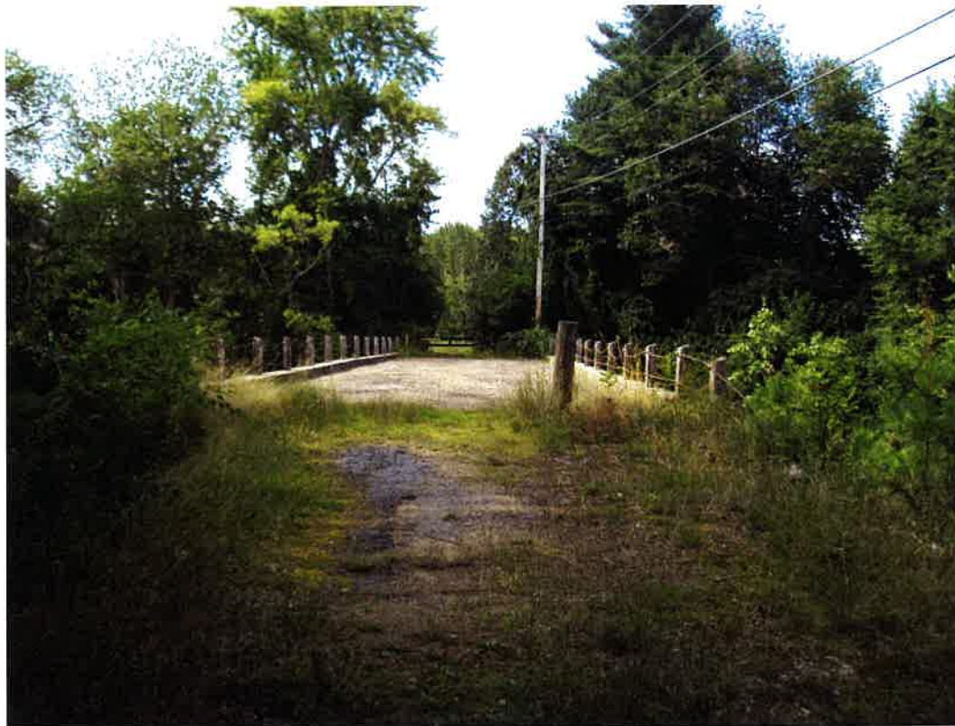
8. View of the second snowmobile trail bridge over the Suncook River from Buck Street Island, facing northwest. 08/15/2019.
