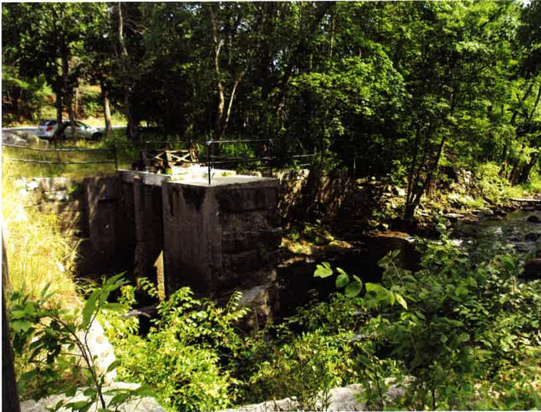
7. View of the former dam penstock controls from the snowmobile trail bridge, facing southeast. 08/15/2019.
