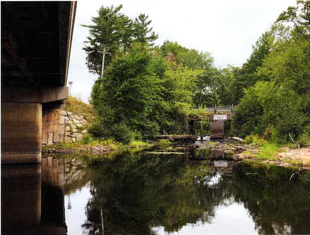
4. Current snowmobile trail bridge over Suncook River, immediately south of the Allenstown Bridge No. 107/098, facing southwest. 09/06/2019.
