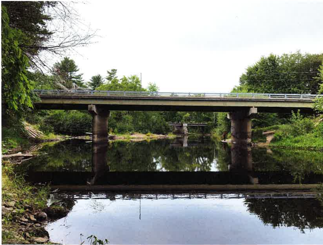
9. View west along the Suncook River, looking toward Allenstown Bridge No. 107/098. 09/06/2019.
