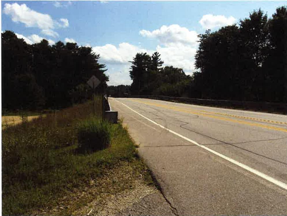
1. Allenstown Bridge No. 107/098 over the Suncook River, northeast railing, facing south. 08/15/2019.
