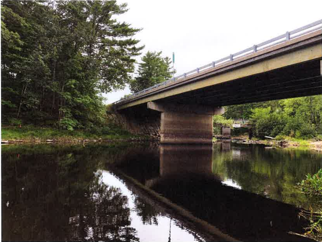
13. View south along the eastern side of Allenstown Bridge No. 107/098. 09/06/2019.
