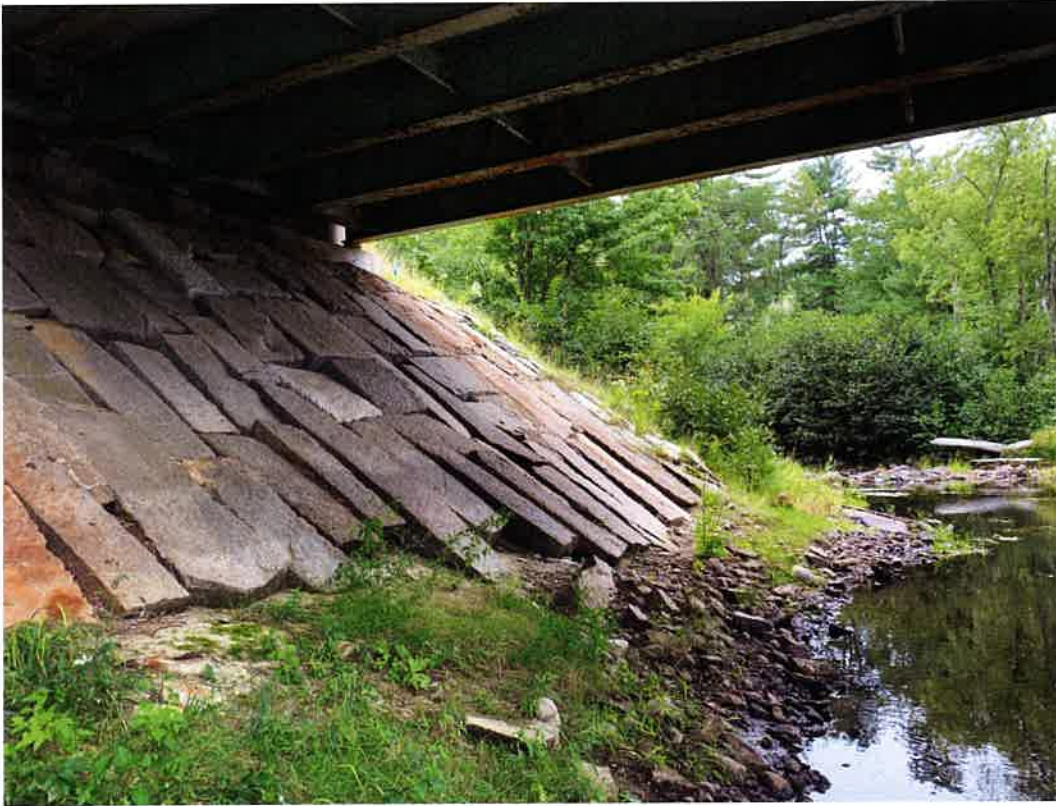
11. View of the southern bridge abutment. 09/06/2019.
