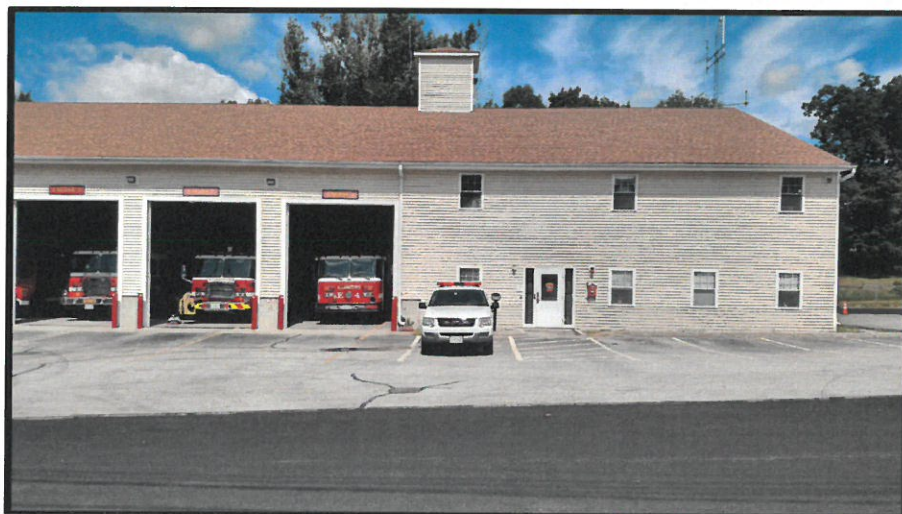
Figure 4 - Ferry Street Fire Station - Front Right
