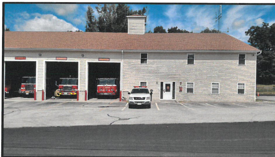
Figure 4 - Ferry Street Fire Station - Front Right
