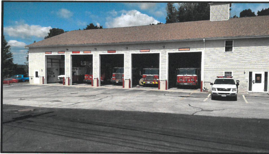
Figure 3 - Ferry Street Fire Station – Front Left
