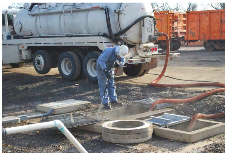
Figure 4. Vactor truck used for Clara maintenance
