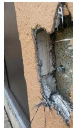
Stucco finish with exposed 1-1/2 inch Styrofoam insulation
