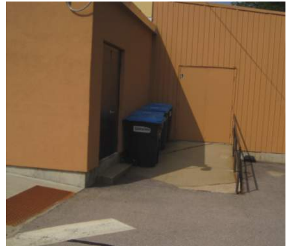
F - Double doors exterior view to Vestibule 139 No landing in front of doors or handrails both sides. If ramp were to be extended to meet code, requirement for landing would interfere with double doors from Storage 138.
