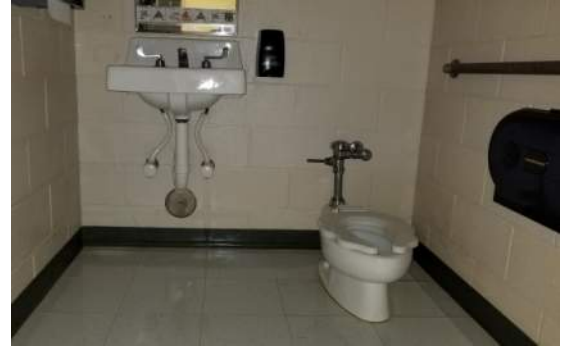
Examples of ADA toilet compartments that have no rear or vertical grab bars
