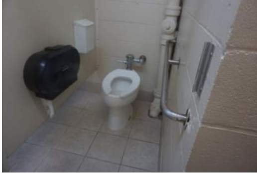
Examples of ADA toilet compartments that have no rear or vertical grab bars
