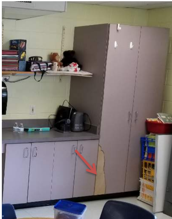
Plastic laminate delamination
