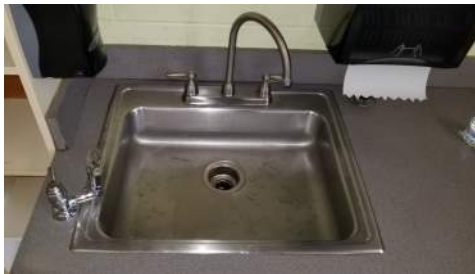
Most classroom sinks have bubbler and per code they must have a separate sink to meet hygiene standards
