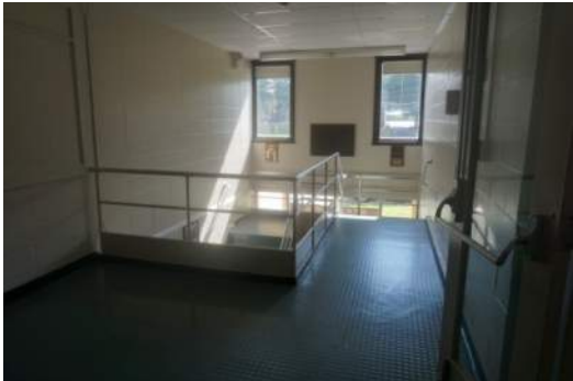
Stair A – handrail termination and guardrail/handrail with balusters along open stair does not meet code.
