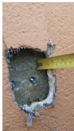
Stucco finish with exposed 1-1/2 inch Styrofoam insulation
