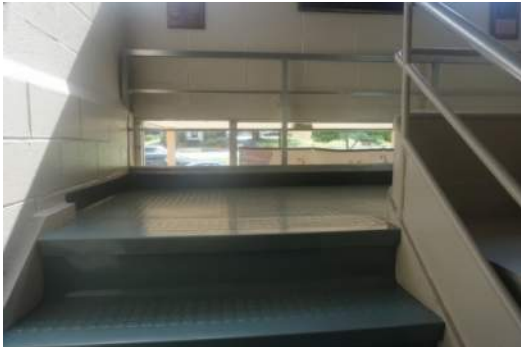
Stair A –guardrail with balusters at landing along open stair does not meet code.
