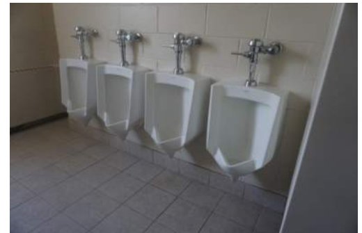
Typical Boys urinals – no ADA code compliant urinals. Require 1 ADA compliant per toilet room in Boys 115 & 213.
