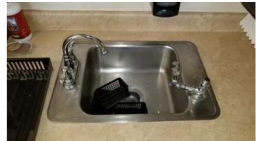
Most classroom sinks have bubbler and per code they must have a separate sink to meet hygiene standards
