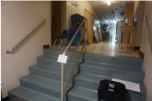
Stair B – handrail termination above and below stairs does not meet code.
