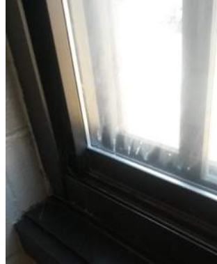
Thermal pane glazing that lost seal
